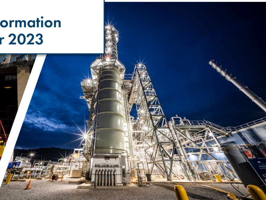
Long Ridge Energy & Power
