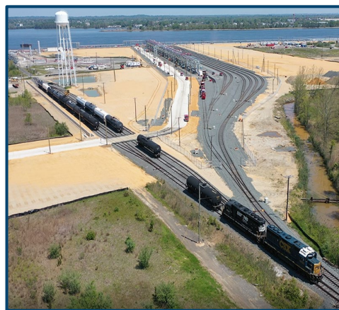
NGL Transloading System
